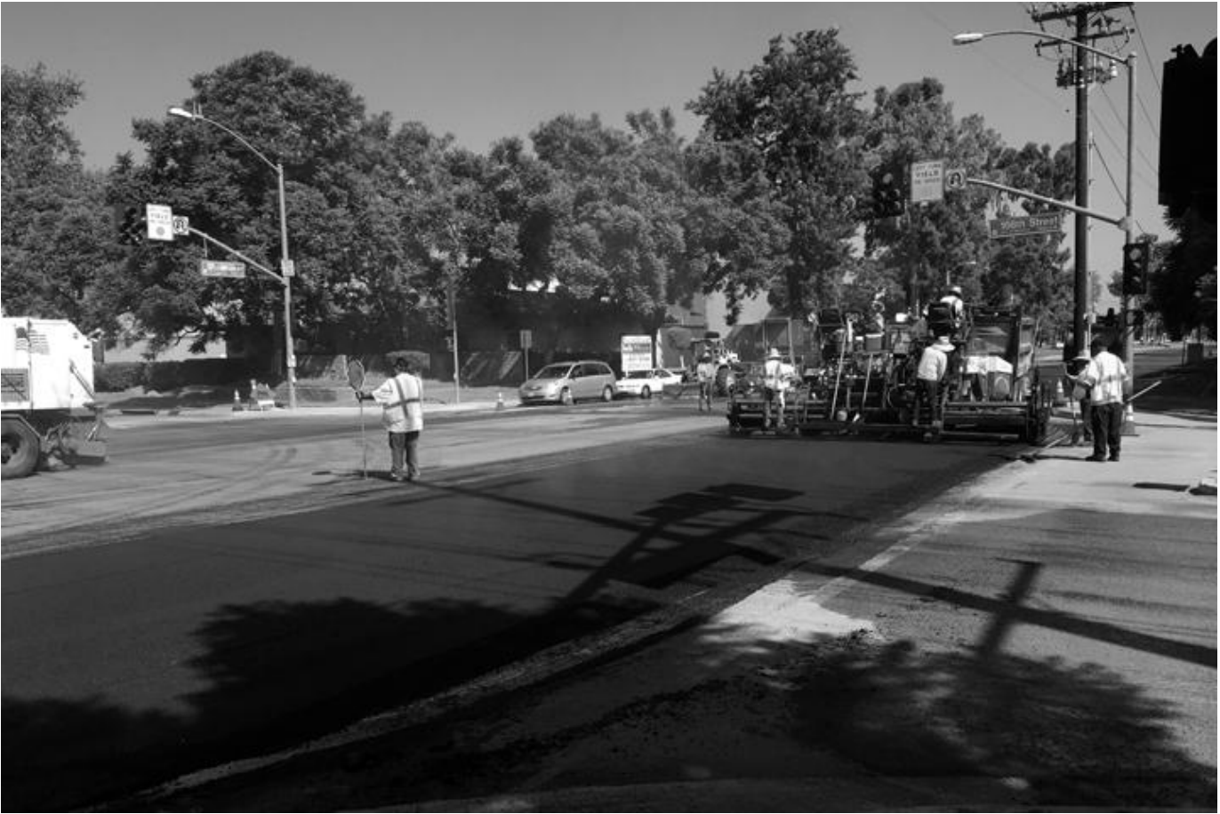
Shoemaker Avenue Rehabilitation
