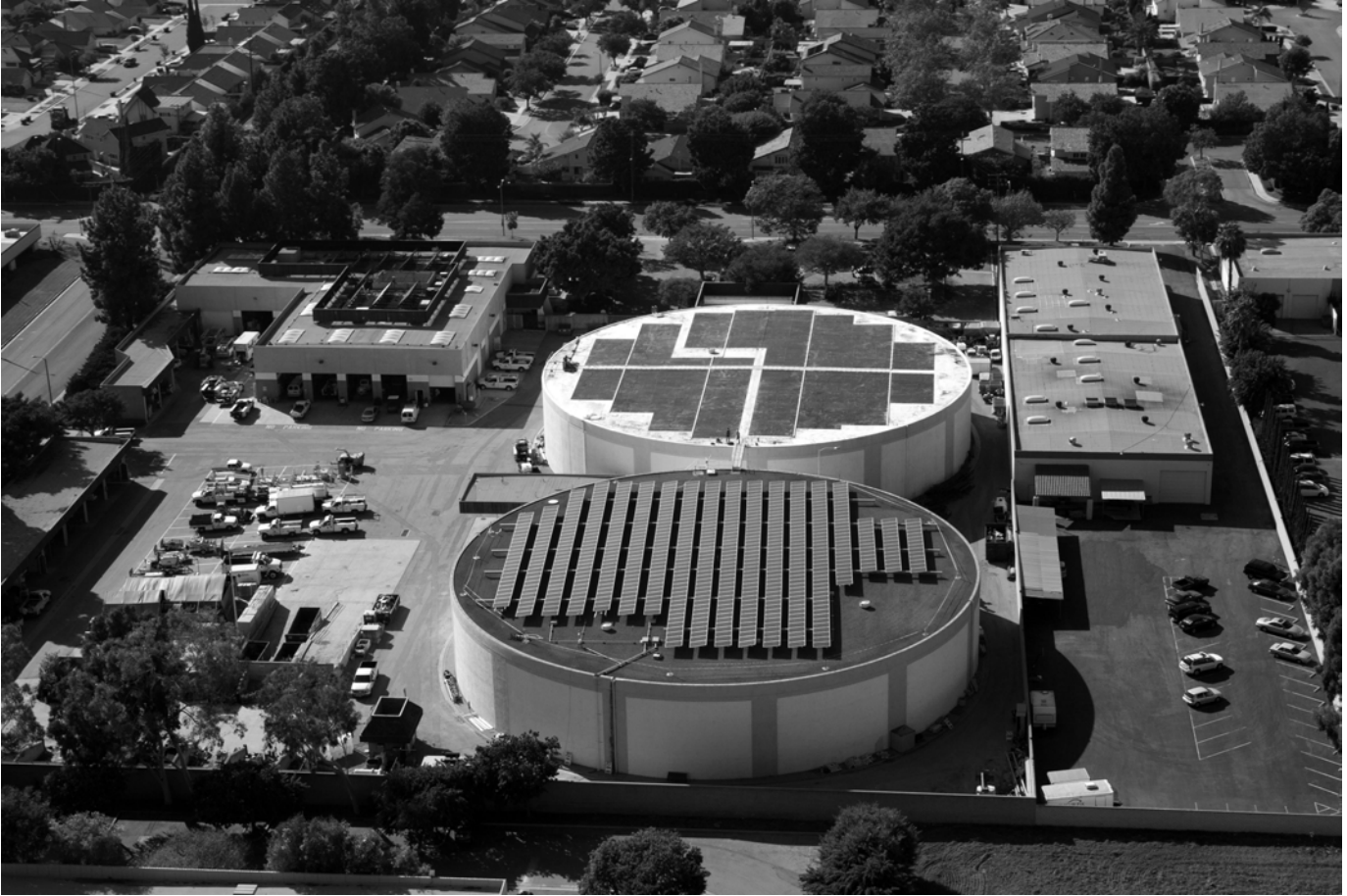
Water Storage with Solar Panels, City of Cerritos Corporate Yard
